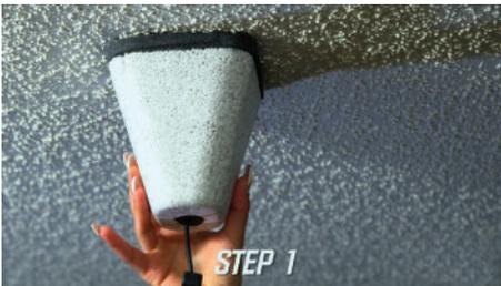
Cover sprinkler heads. Bed Bug Heat Doctor/PrevSol is not liable for any damage if sprinkler heads are not covered. We recommend using an outside faucet cover available at a local home improvement store. It keeps your sprinkler head 30 degrees cooler than the room temperature.
